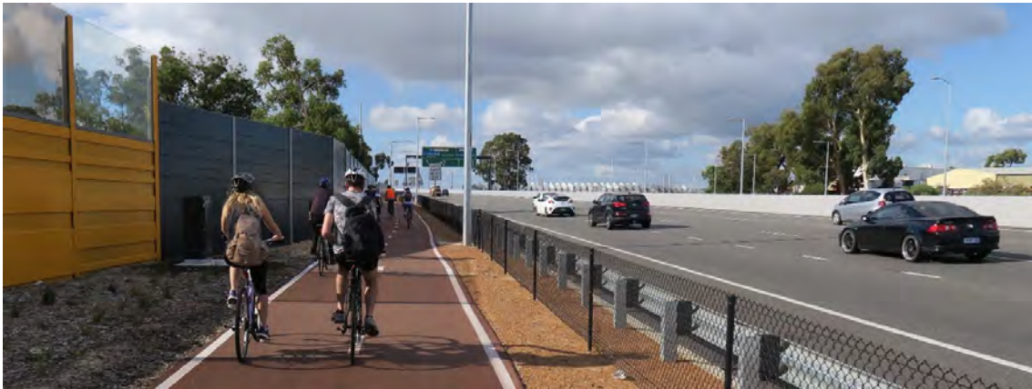
Above: Perth major infrastructure investment for the Gateway WA project provided an opportunity to build high quality shared paths. Photo by Stephen Hodge shows Leach Highway near Perth Airport. Perth 2017.
